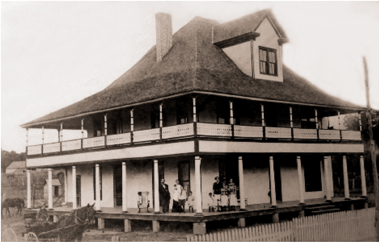
CHAPMAN HOUSE AFTER THE SECOND STORY WAS ADDED. DATE IN CITY HALL SAYS 1910 BUT IT IS PROBABLY LATER. SOURCE: HOLLYWOOD CITY HALL
