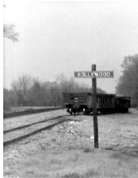
STATION CROSSING SIGN IDENTIFYING HOLLYWOOD SOUTH OF TOWN. SOURCE: CITY HALL
