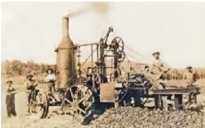
DITCHING MACHINE WHICH PREPARES A FIELD FOR LAYING DRAINAGE TILES. WILLIS NEHER IS THE ADULT IN THIS PHOTO. FROM THE HUNTSVILLE TIMES AND FROM THE PAUL MACHEN COLLECTION
